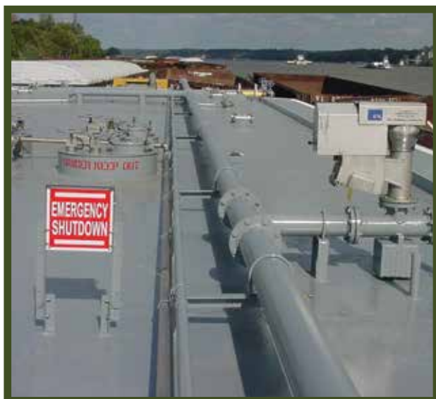
Superac 6" High Velocity PV valve Model II - Mounted on collapsible piping next to Emergency Shutdown (EMS-001) sign with stainless steel frame (EMF-001).
