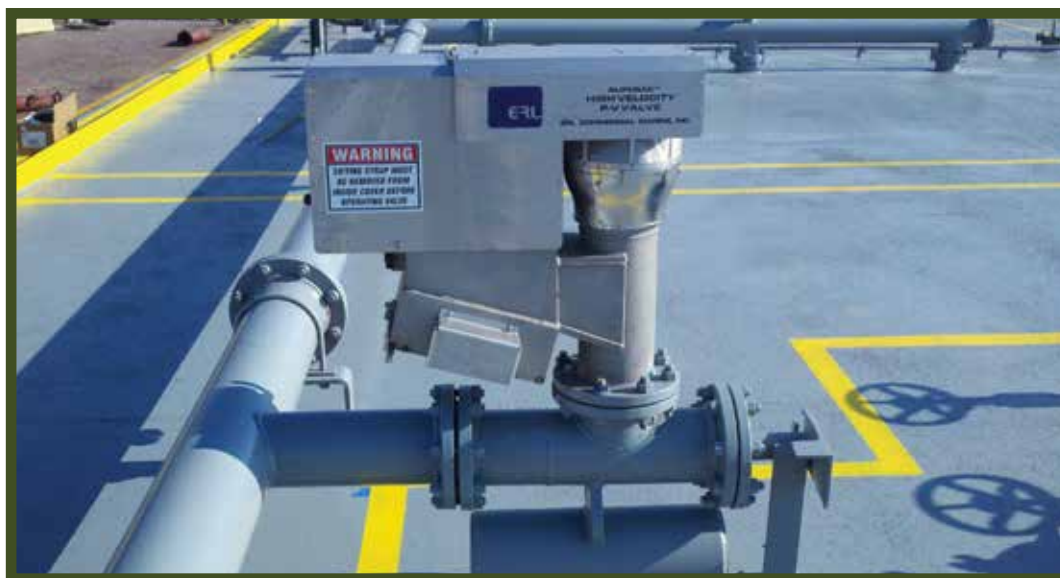
Superac 6" stainless steel High Velocity PV valve Model II - mounted on collapsible piping.
