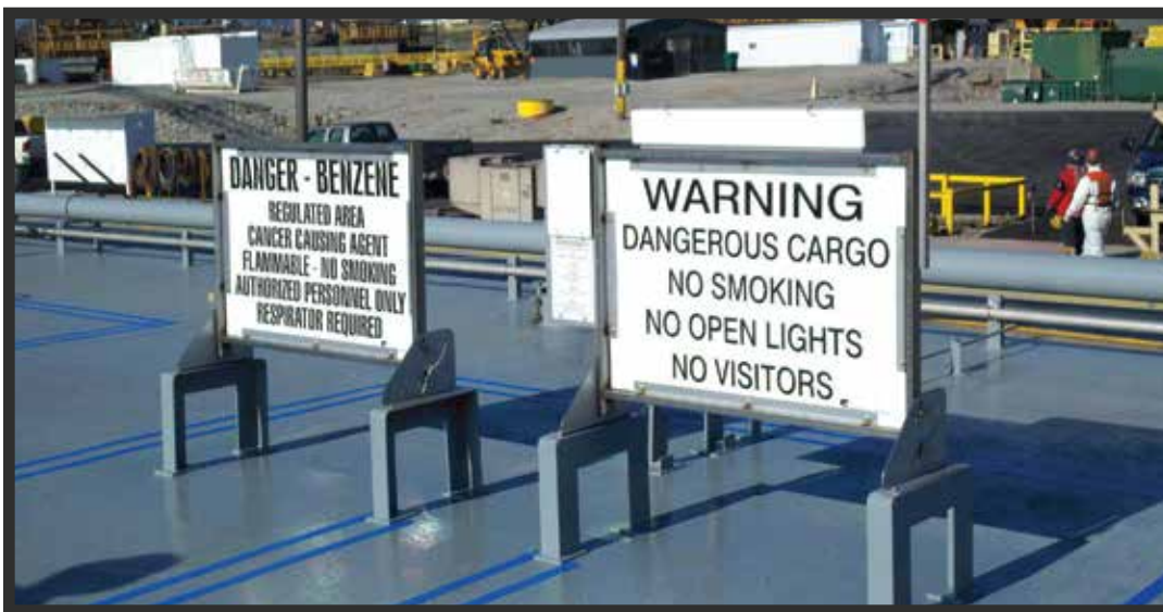
Warning Dangerous Cargo Sign with Frame containing CGS sign on top CIC sign and NOT sign on side mounted next to Danger - Benzene Sign with Frame.
