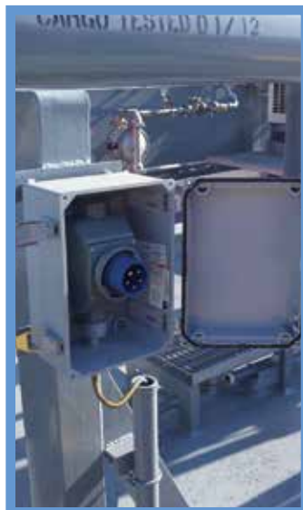
BTS-1 Barge-to-Shore Connector with BCS-001 located on outside of Hubbell weather tight box.
