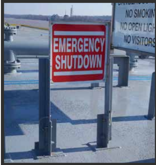
Emergency Shutdown sign and Frame mounted next to Warning Dangerous Cargo Sign and Frame.
