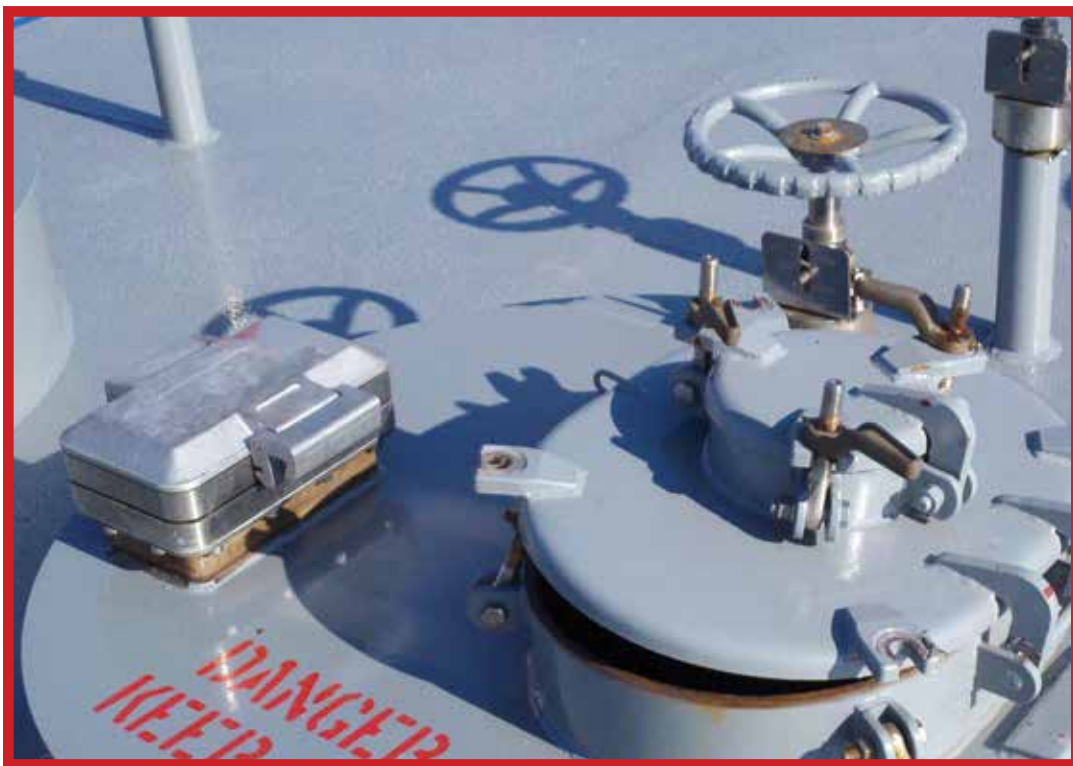
Full View Model SGM-1™ Sight Glass - weather covers closed - mounted on expansion domes.
