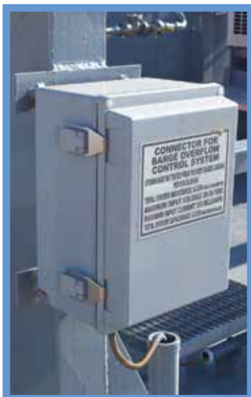
BTS-1 Barge-to-Shore Connector with BCS-001 located on outside of Hubbell weather tight box.
